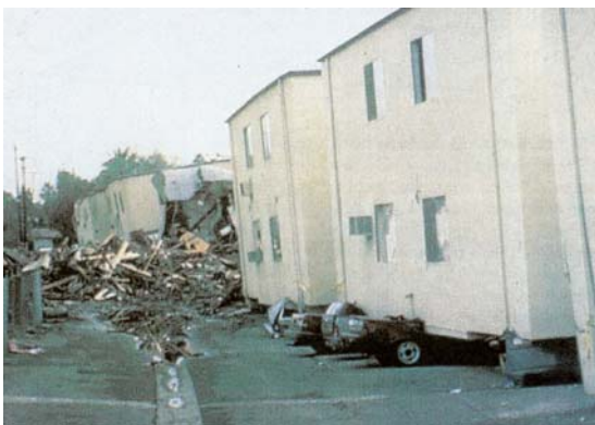
Figure 1a. Example of soft story collapse.
