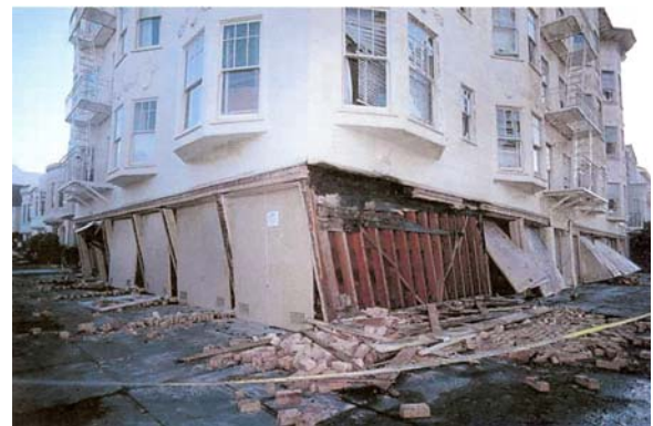
Figure 1b. Example of soft story collapse.
