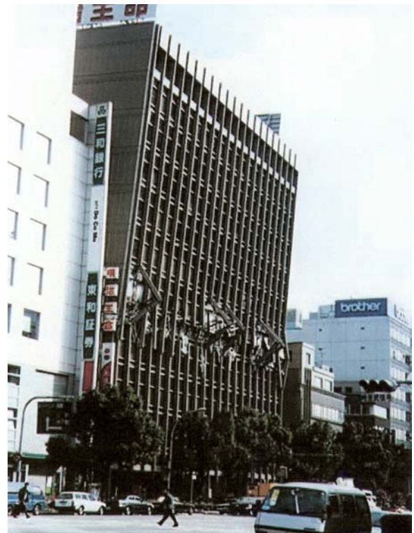
Figure 1c. Example of soft story collapse.
