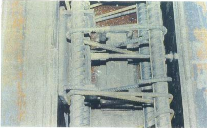
2.25 BSF units placed on side and in bottom.
