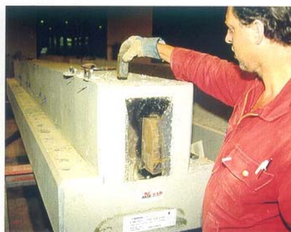
4.42 Placing of lock-pin.
