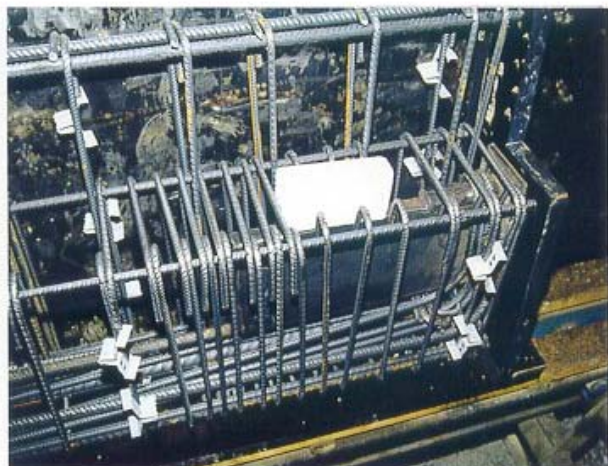
3.34 Removeable polystyrene in upper face of beam
