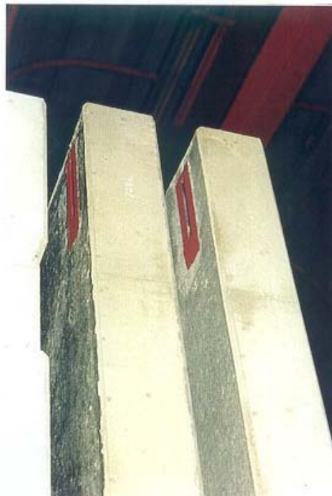
4.50 Wall element with support for beam.
