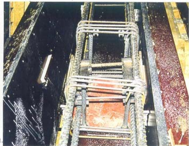
2.22 The guiding knives ensures accurate positioning of the BSF-units.
