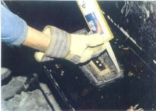
2.19 Guiding knife in bottom of form sealed with silicone.
