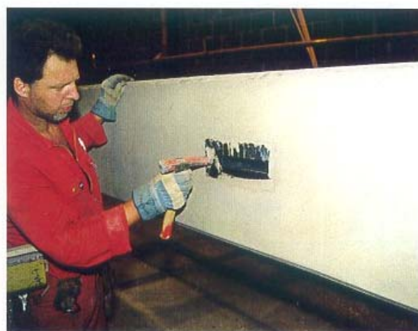
4.40 Cleaning column unit.
