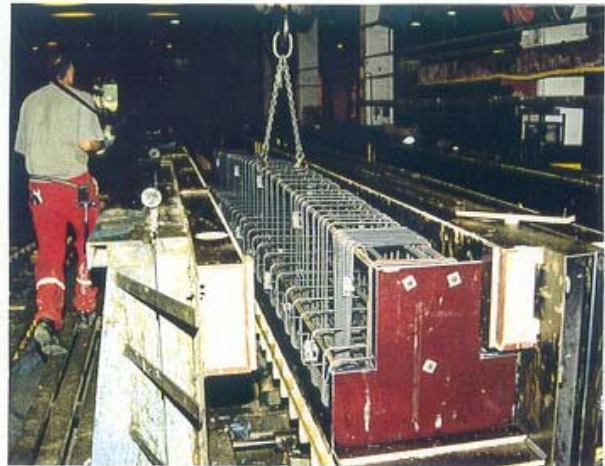
3.32 The complete reinforcement hoisted into final position in form.
