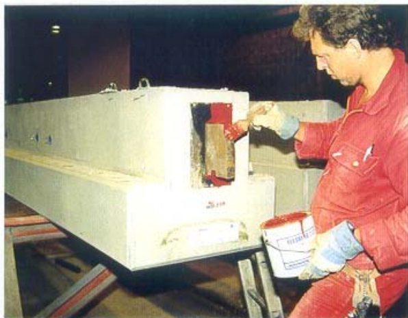
4.43 Some customers wants painting. (-beam)
