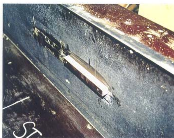
2.16 Guiding knife in plywood form.
