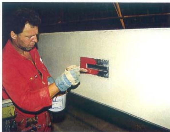
4.44 Some customers wants painting. (-column)
