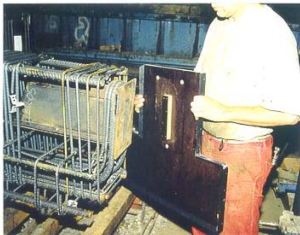
3.29 Endplate with guiding knife, centre-beam.
