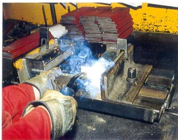
2.9 Double column units welded in jig.
