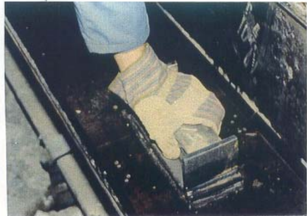
2.20 The column unit is pressed into position. Watertightness ensures underpressure.
