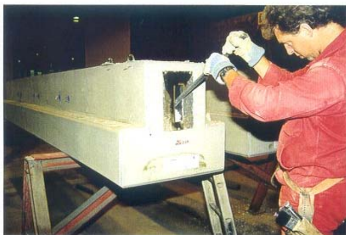
4.37 Removal of polystyrene.
