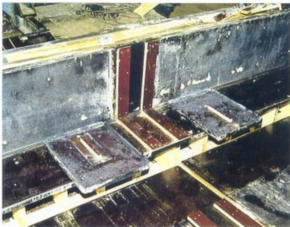
3.33 Placing of end plates in middle of form.
