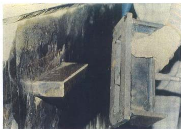
2.15 Guiding knife spot welded to form.
