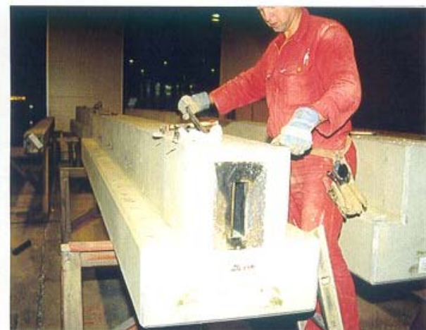
4.36 Removal of polystyrene.
