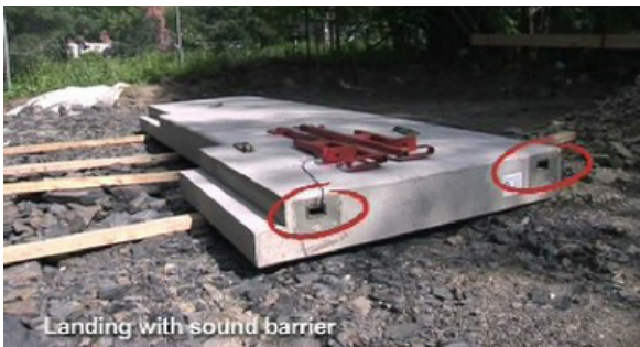
M1: Landing with TSS and rubber box.
