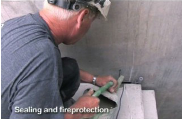
M13: Fill the gap with mortar
