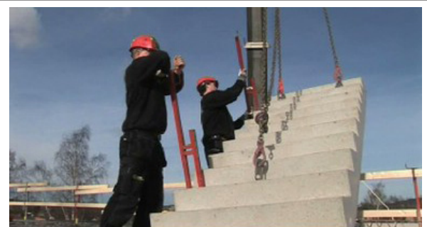
M18: Placing temporary railing to the stair.
