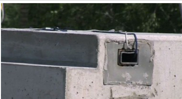
M3: Place the rope on the top of the landing before Lifting.
