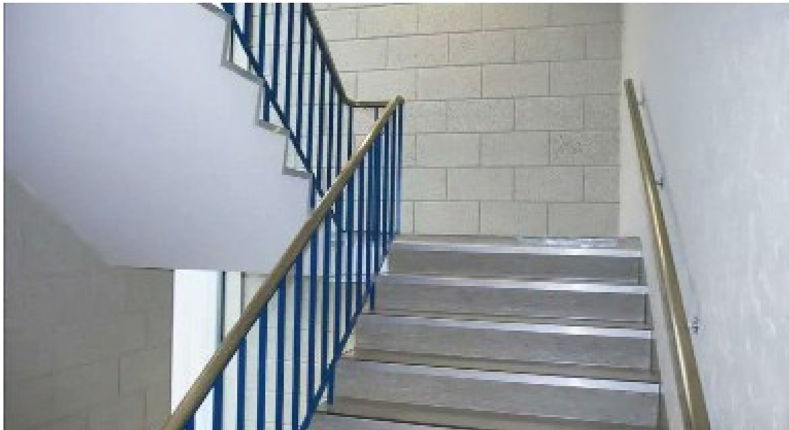
M25: The stair is finish.
