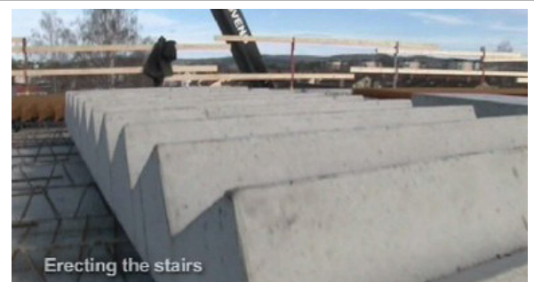
M16: Stair ready to be erect.
