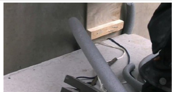
M10: The sheathing list in the right position.
