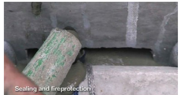
M14: The mortar are also fireproofing the unit.
