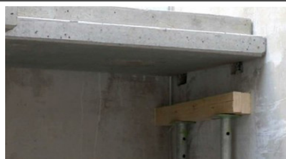
M6: Landing almost in the right position.
