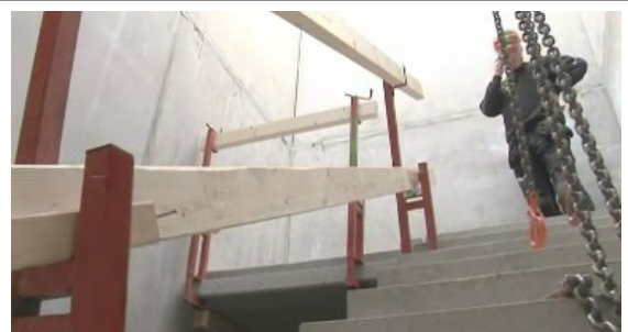
M24: The landing and the stair are finish. Ready for the next floor.
