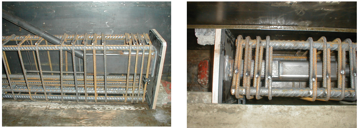
Figure 6. The reinforcement cage in the test beams.
