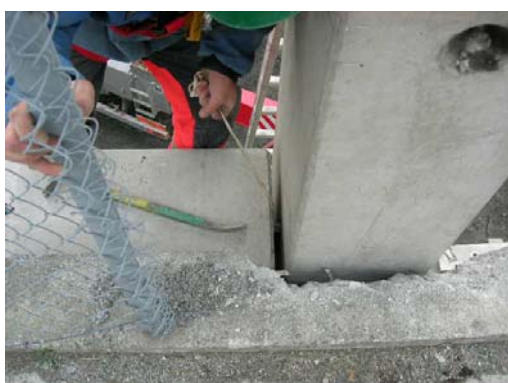
E5. Pull the double rope, until the knife is in the right position.
