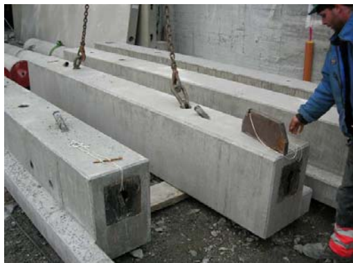
E1. Preparation of the beam before lifting. Safety rope is rearrange to be able to pull out the knife.
