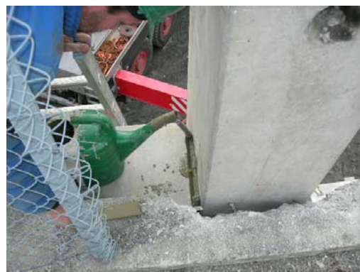
E8. Filling the joint with mortar (eg. "Nonset").
