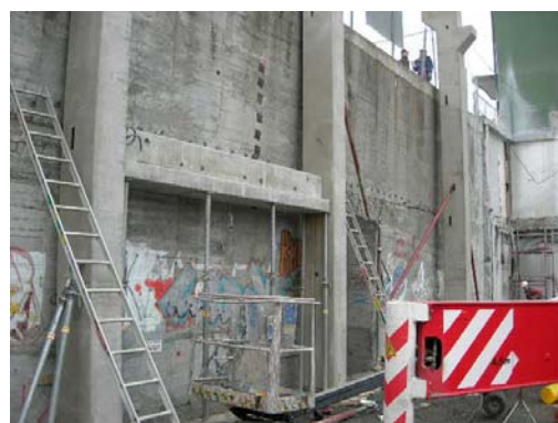
E4. The beam is lifted in place, and supported.
