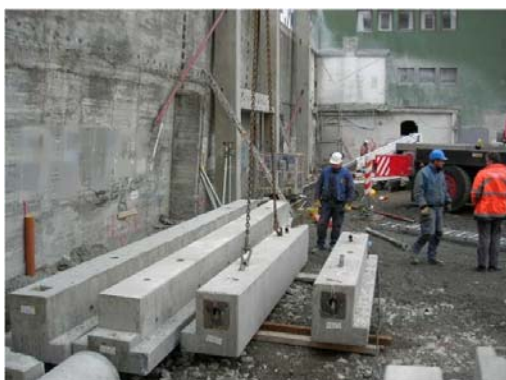
E3. Mounting the lifting hooks.
