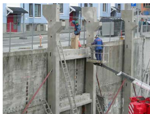
E6. Insert the backing in the joint between the beam and the column.
