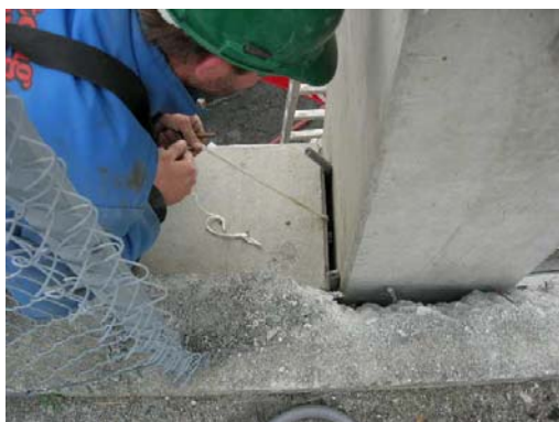
E7. Cut the rope, and pull it out.
