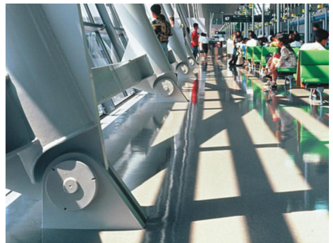
Figura 45 – Cerniera cilindrica, Kansai International Airport (Osaka)
