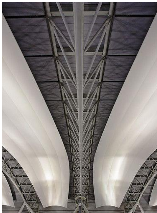
Figura 33 – Corrente inferiore CHS unico, Kansai International Airport (Osaka)
